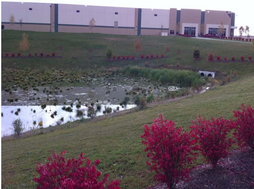
Post Construction Storm Water Management Basin
