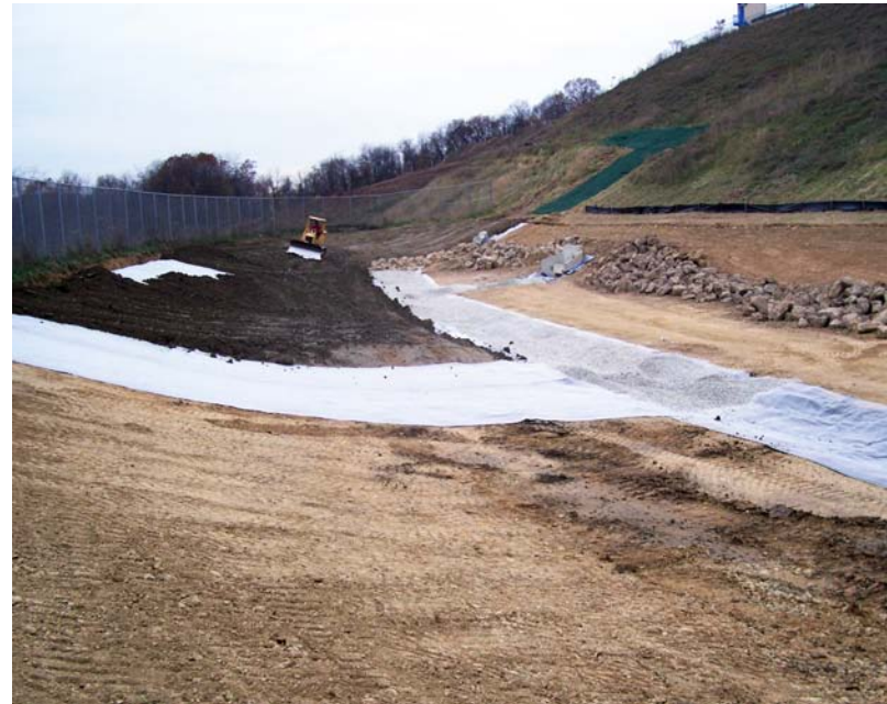
Detention Pond Reconstruction
